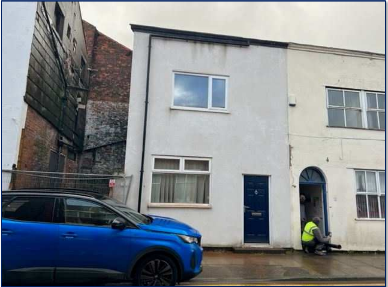
St Wilfrid Street Frontage
