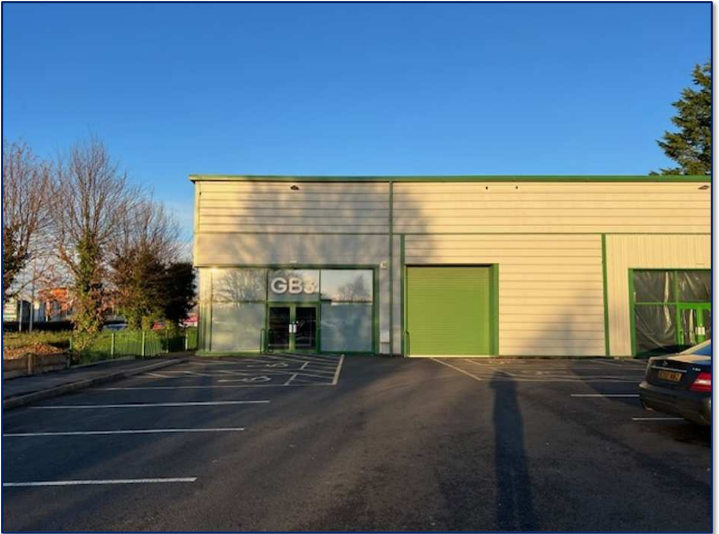
Indicative photograph showing the installation of a new roller-shutter door in the front elevation.
